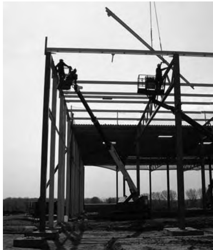
Fig. 5: Aerial work platforms
