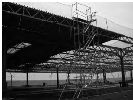
Fig. 13: Freestanding stair towers
