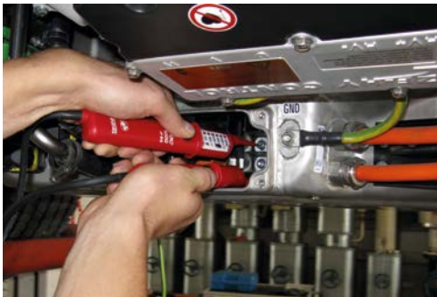
Figure 3: Verification of the non-live state
